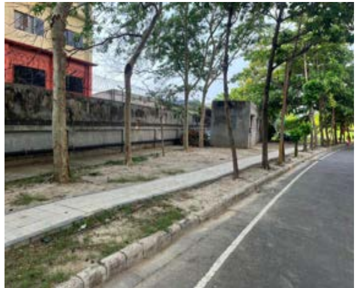
From the new Pump House upto Tower 5 Gas Station
